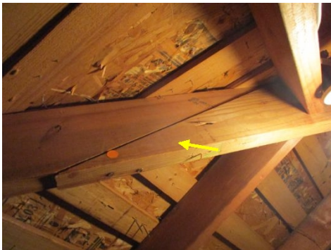
There are several cracked rafters visible in the attic area; see dots.
