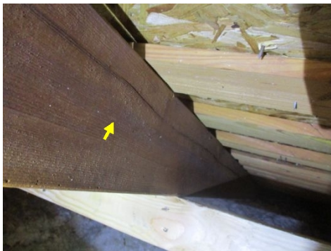
There are two areas that appear to have had additional horizontal support added, I am unable to verify if additional vertical supports are needed at those locations.
