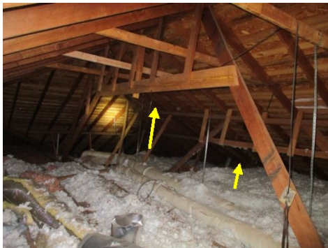
There are two areas that appear to have had additional horizontal support added, I am unable to verify if additional vertical supports are needed at those locations.
