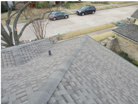
Some nails need to be sealed at the rooftop to prevent them from rusting.
