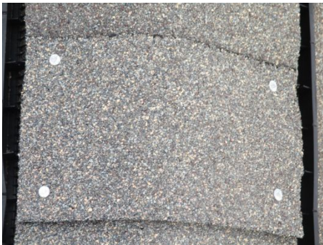
Some nails need to be sealed at the rooftop to prevent them from rusting.
